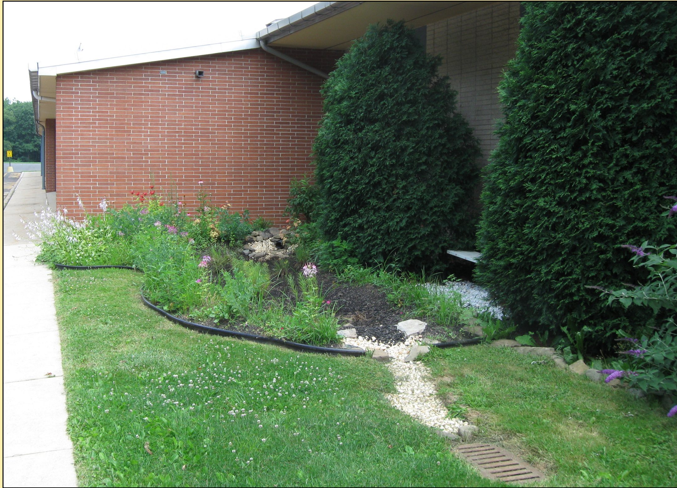
Rain gardens can be used to collect water from rooftops as shown above at Blair Mill Elementary School in Horsham Township, Montgomery County.
